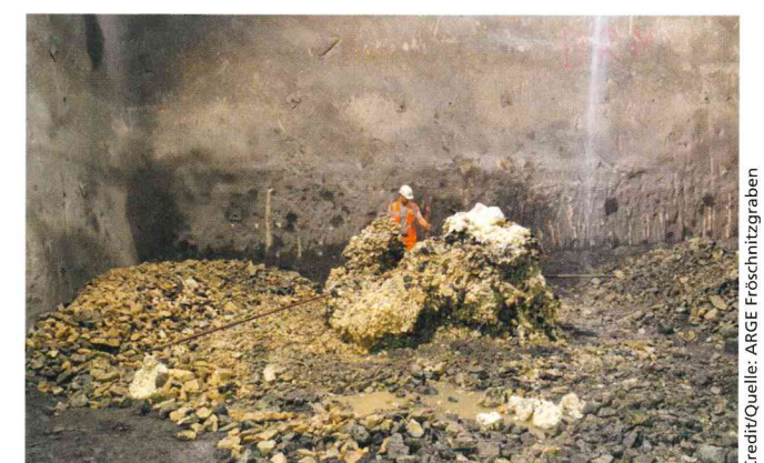
4 Injection test 2 in muck pile, this time with relatively blocky material Injektionsvorversuch 2 in Haufwerk, diesmal in relativ blockigem Material
